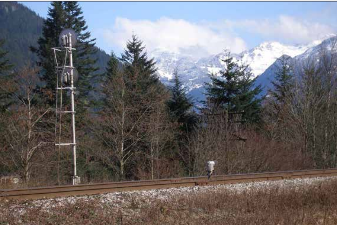
A RAILROAD TRACK NEAR THE QUOCAHALLA HIGHWAY
