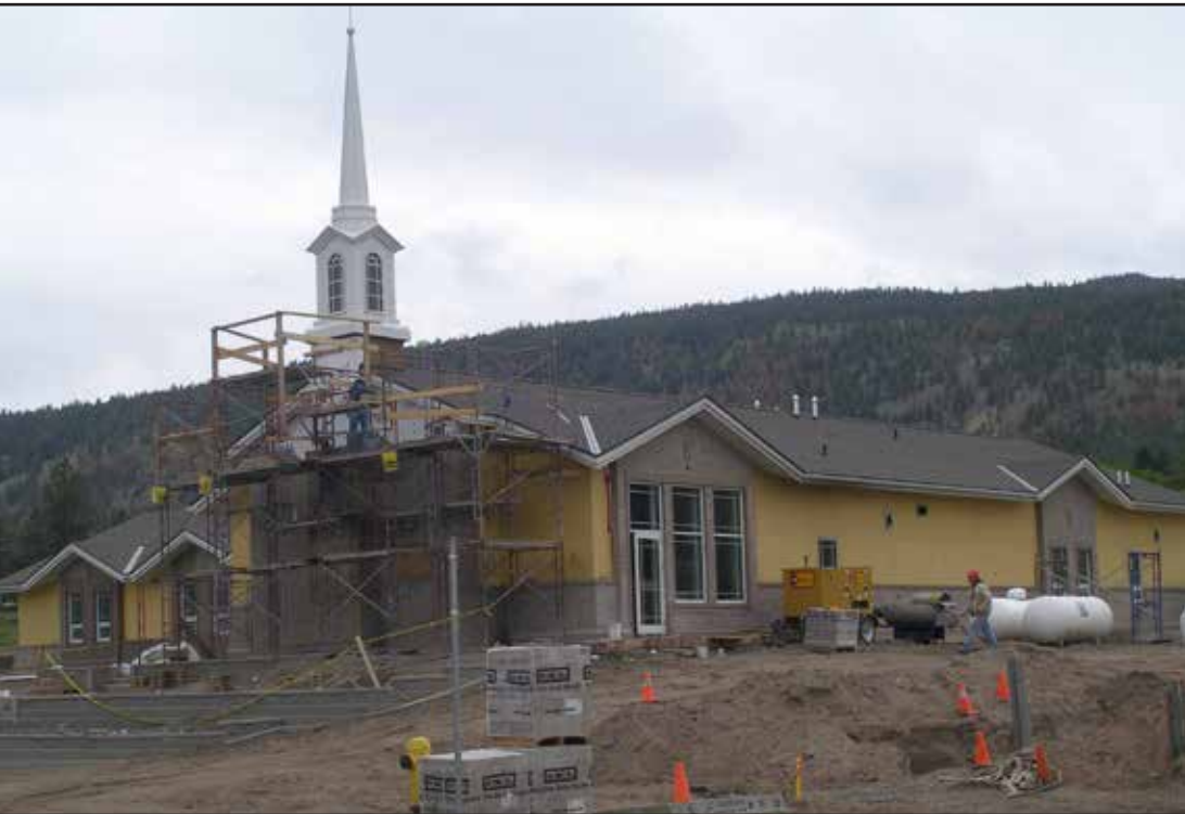
MERRITT CHAPEL UNDER CONSTRUCTION
